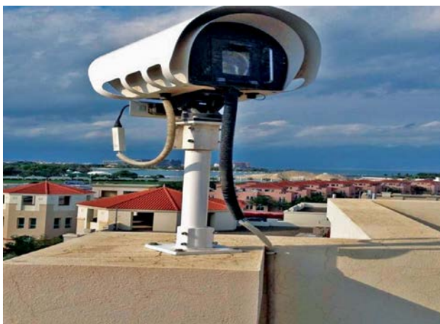
Figure 6. UOWD FSO installation with mounting bracket
